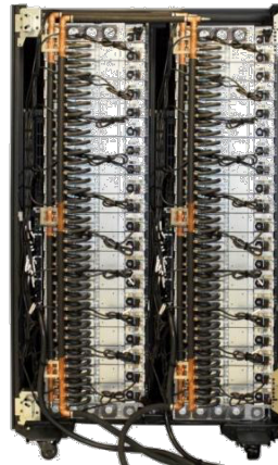
iDataPlex DWC Rack w/ water cooled nodes (rear view of water manifolds)
