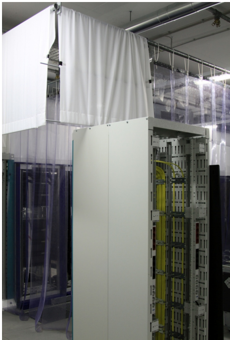
Implementation of a cold and hot aisle containment which is compatible with the argon fire extinguishing concept
