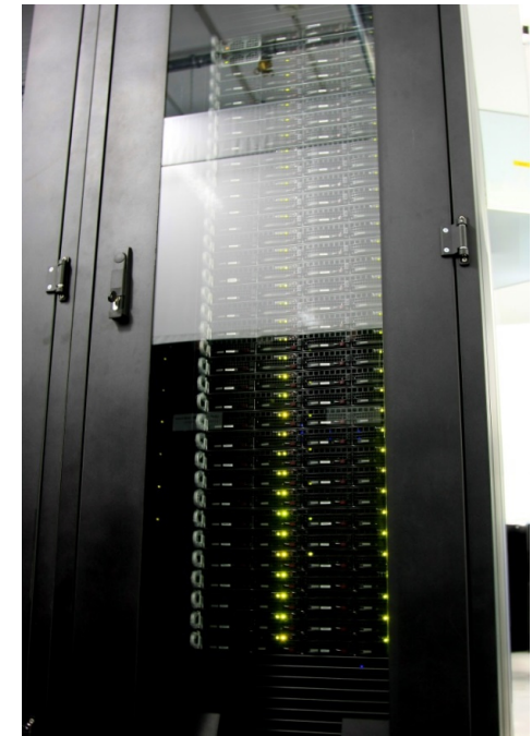
Installation of a room neutral and direct liquid cooled rack solution for very high power densities > 15 kW per rack
